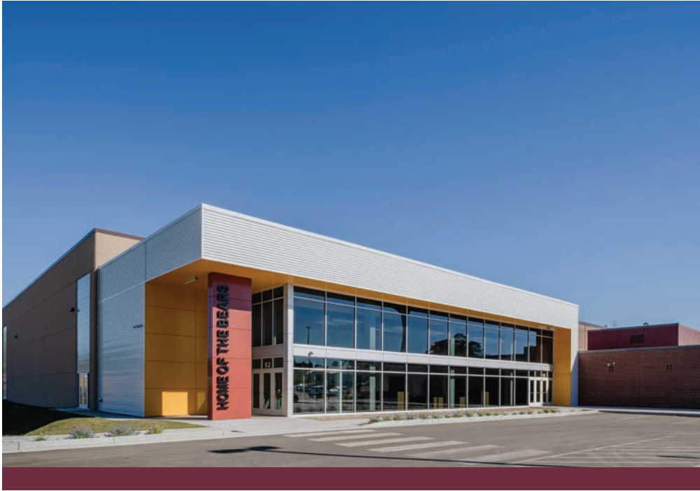
Exterior view of the Barron High School competition gymnasium addition
